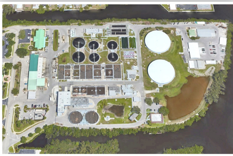
The City of Naples Water Reclamation Facility (WRF) transforms wastewater into reclaimed irrigation water, making for lush lawns and green golf courses during Florida's dry season.
