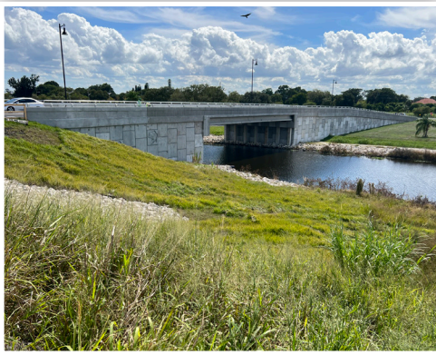
The newly constructed C-21 bridge in Clewiston will allow boaters to access the west side of the bridge from Lake Okeechobee.
