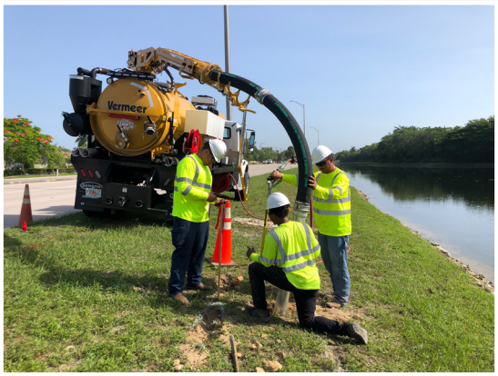
Our surveying and mapping team recently acquired the newest line of Vermeer's high-capacity, 4-wheel drive, diesel truck-mounted vacuum excavation to perform SUE services.
