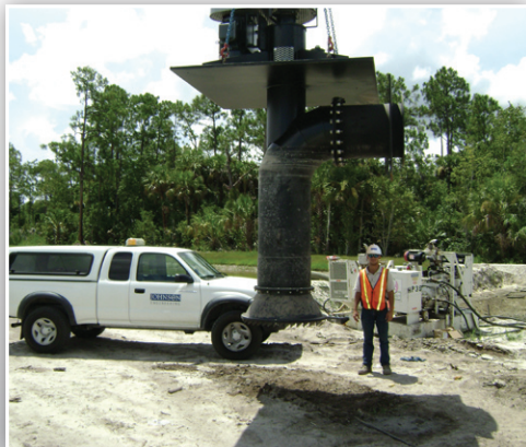
Erik Howard onsite for the installation of dual 12,000 gpm pumps for a pump station to rehydrate existing wetlands for the Lely Area Stormwater Improvement Project (LASIP).
