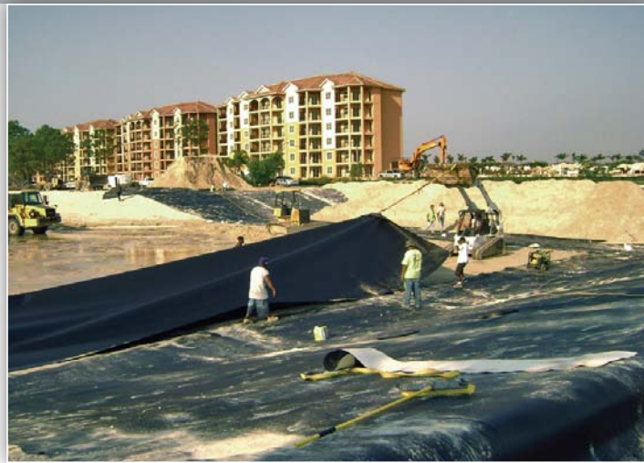
Installation of the 60 mil thick textured HDPE liner in the constructed lake.
