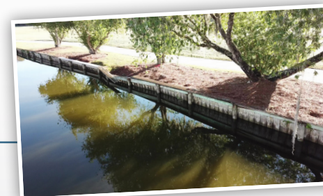
Assessing lake bank erosion
