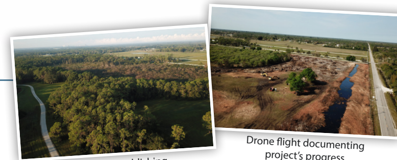
Drone flight establishing existing conditions, Drone flight documenting project's progress
