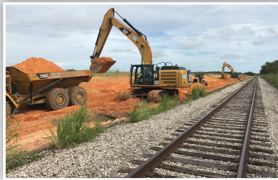
Earthwork was a challenge given the existing terrain. Over 30,000 CY of soil was moved in a matter of weeks.
