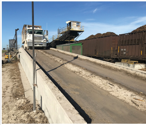
The SCFE's Childs Siding loading facility in Lake Placid will get a new loading ramp, like that above, to easily load freshly harvested sugarcane into waiting rail cars so that it may be hauled to U.S. Sugar's mill in Clewiston.
